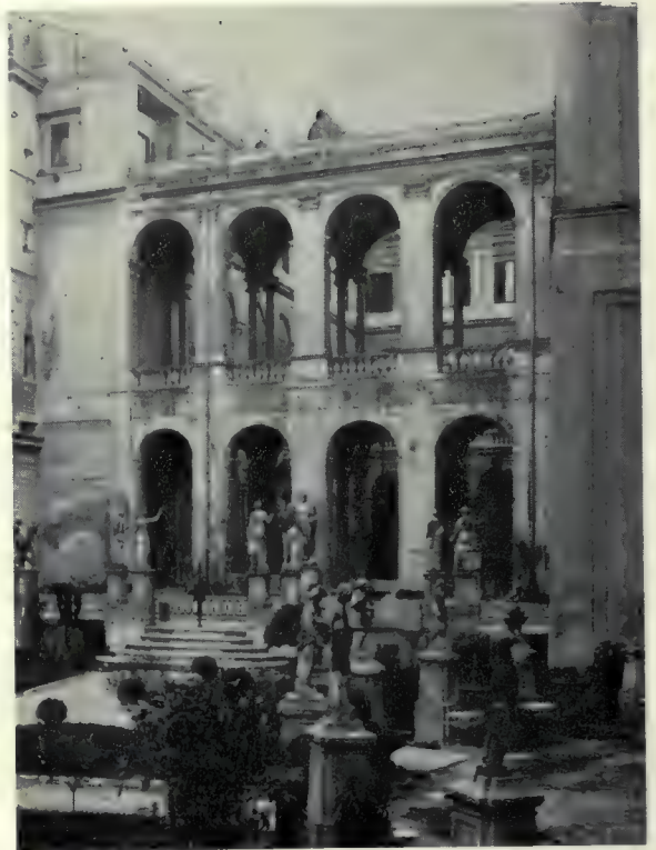
60. - Palazzo Borghese. Bridge loggia from garden.
